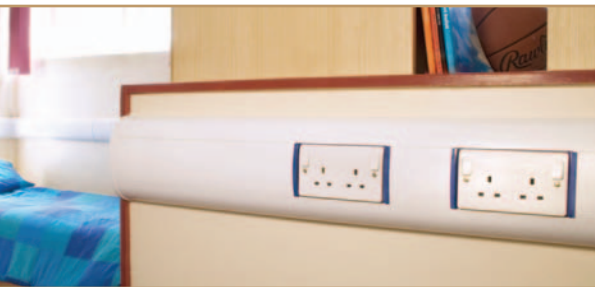
Blue accessory boxes installed within trunking at Old Swinford Hospital School
