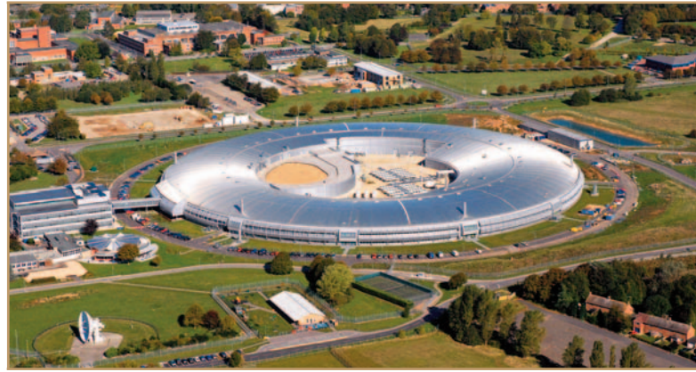
Perimeter Trunking with Electromagnetic Shielding installed within The Diamond Synchrotron, Oxfordshire.
